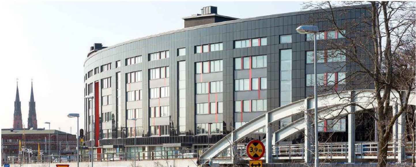
COLD FAÇADE BIPV SOLUTION, FRODEPARKEN (UPPSALA, SWEDEN) (ARCHITECT: WHITE ARCHITECTS )
