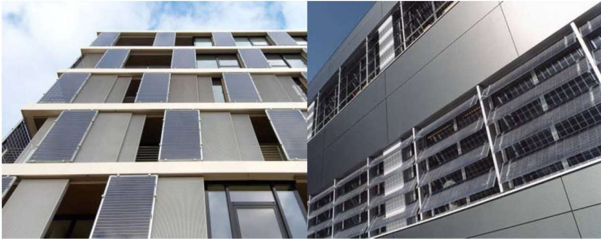
Fig. 3.B.28: solar shading solution: Left: Colt Ellisse PV sliding shades at Company HQ, Bitterfeld-Wolfen, Germany, © Colt, Right: Keuringsdienst, Eindhoven, The Netherlands, Yanovshtchinsky Architekten: using Colt Shadovoltaic as shading device, © Colt.
