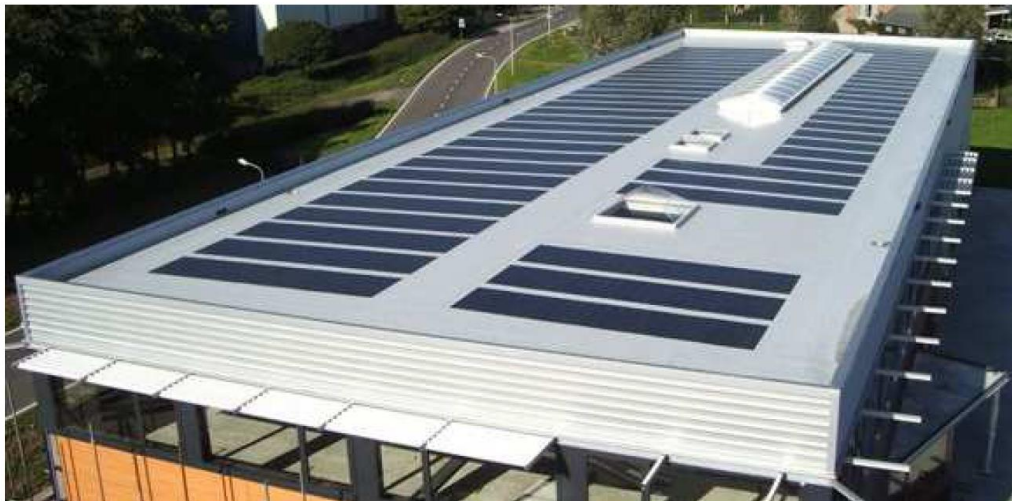
PV MEMBRANES EMBEDDED IN A FLAT ROOF COVER (SOURCE: WEKA DAKSYSTEMEN).
