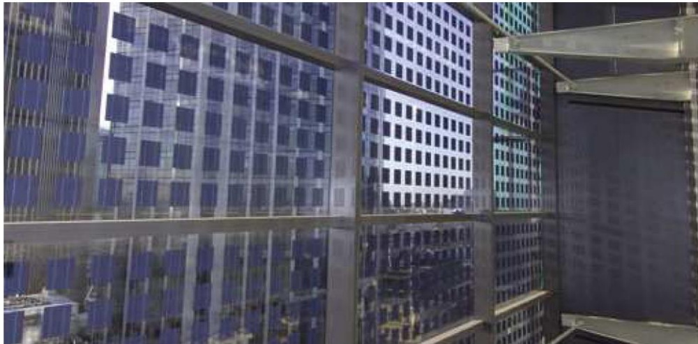
THE "HERON TOWER" IN LONDON WITH THE SEMI-TRANSPARENT DOBLE SKIN -BIPV FAÇADE (PICTURE: P. BONOMO).
