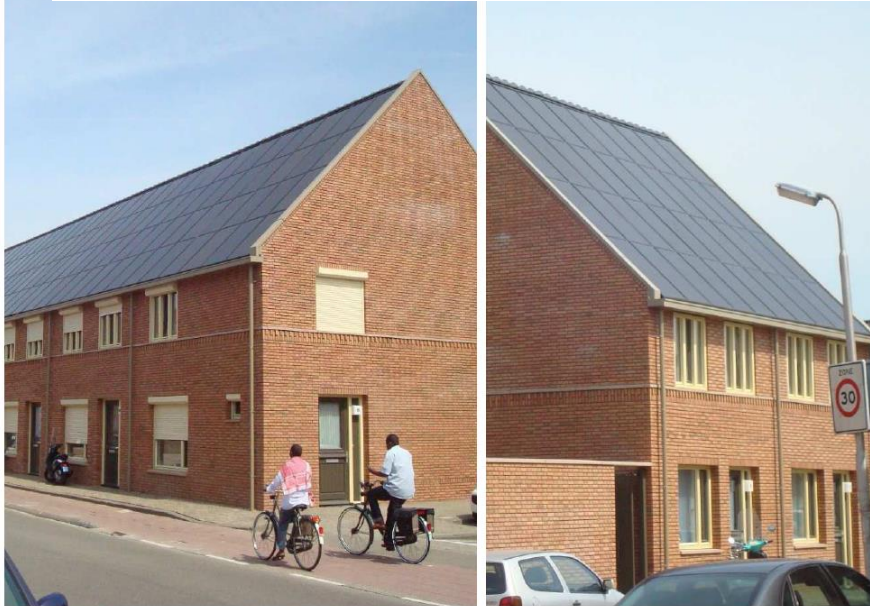
SCX SOLOROOF AS BIPV FULL ROOF SOLUTION (TILBURG, THE NETHERLANDS), 75 TERRACED DWELLINGS
